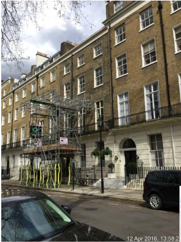
Photograph 1: Application property (with scaffolding in front)
